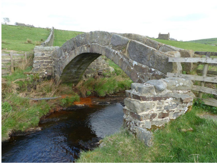
Figure 2 Grade II listed packhorse bridge over Colden Water near Hebden Bridge, Calderdale.
