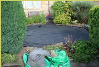
This small project in Mytholmroyd uses recycled plastic for both the weed barrier layer and edging for a gravelled area.
